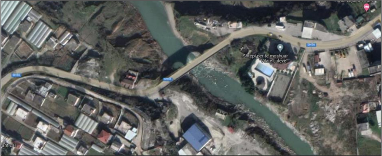
Figure 8: Beshiri Bridge over the Erzeni River – top view
