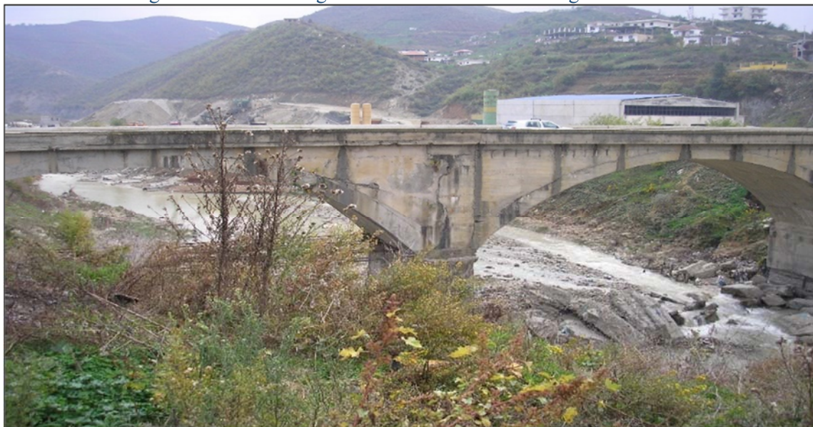
Figure 7: Beshiri Bridge over the Erzeni River – side view
